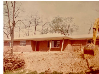
Green home under construction in 1972-73
